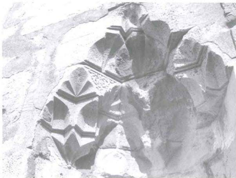
69 Muqarnas niche on the north side of the west porch of Hagia Sophia
